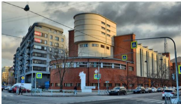
Figure 6. The Power Plant (2018 photo).
