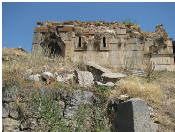
Figure 1. Neghuts monastery: view from the south.
