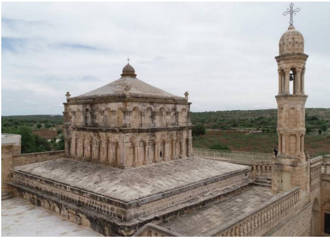
Figure 3. Exterior view of El 'Adra church: looking northwest (from: https://pg.world/rus/user/public_tours/view?id=60922712f332430e73523075 ).
