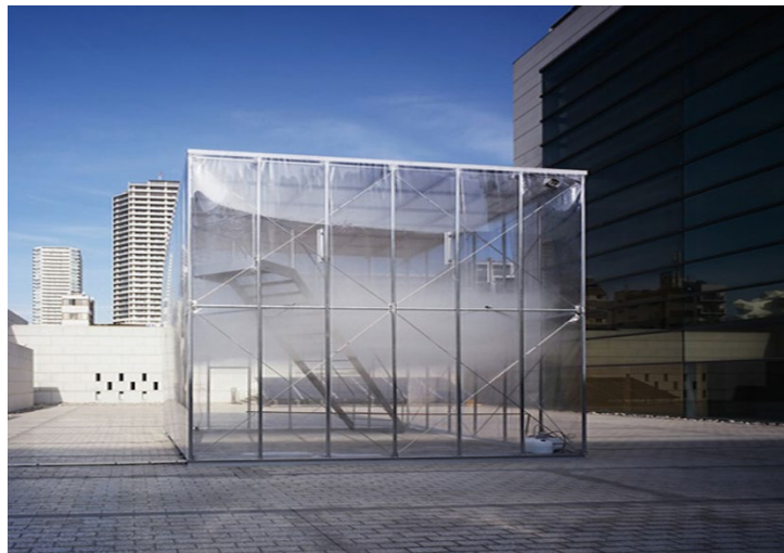
Figure 3. Tetsuo Kondo (architect): "Cloudscapes" in the Museum of Contemporary Art in Tokyo, Japan.
